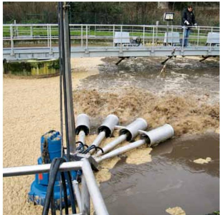
Figure 43: Venturi system for injecting oxygen into stabilisation ponds
