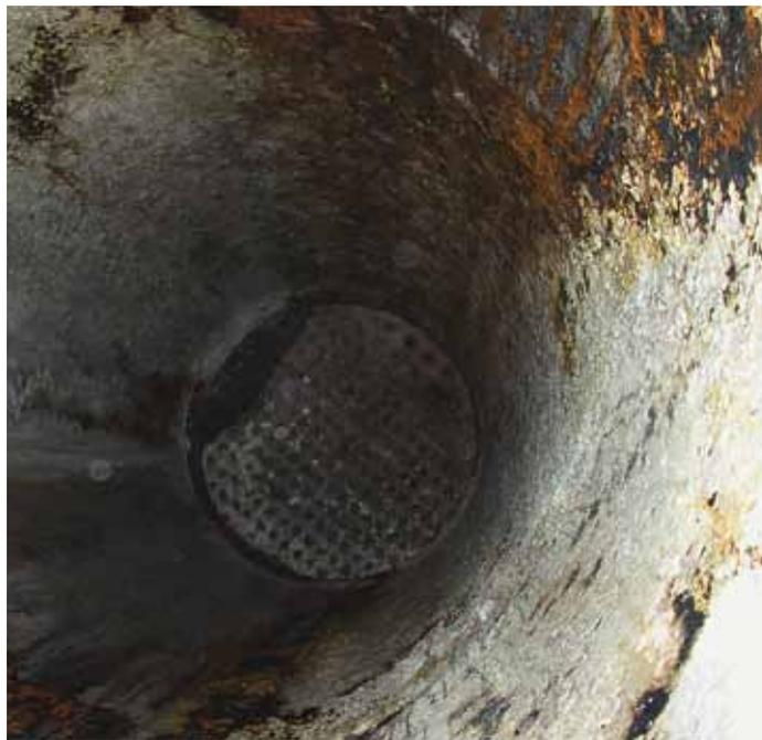
Figure 33: Corrosion caused by ammonia salt deposits
