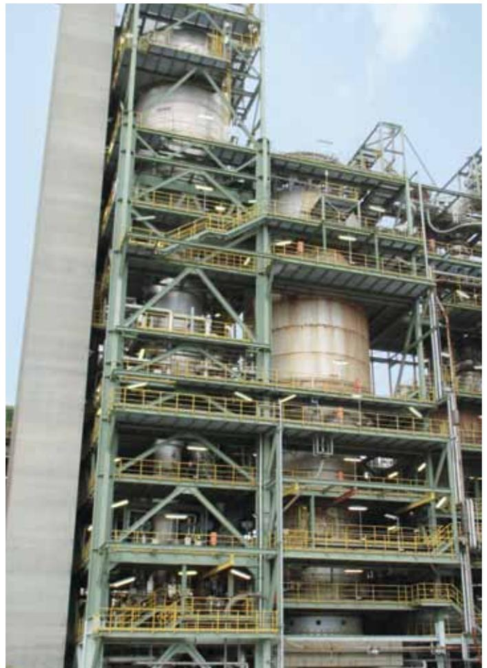
Figure 37: FCC unit in a German refinery (with kind permission of TOTAL Raffinerie Mitteldeutschland GmbH)
