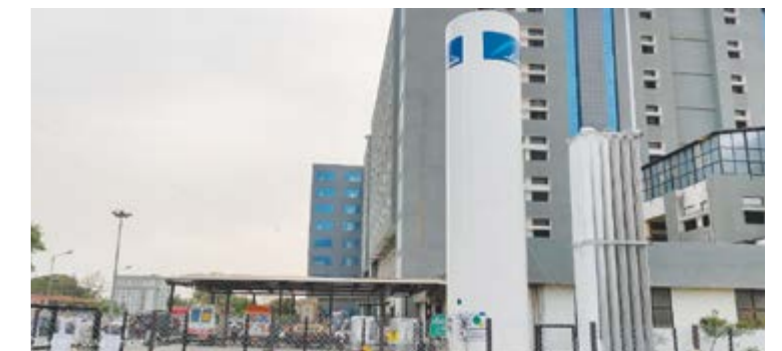
Medical oxygen installation at various partner hospitals to ease the supply of oxygen. Among others, Linde recently installed a 20 KL tank at GMERS Medical College, Junagadh, Gujarat.
