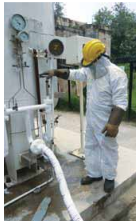
Decantation of LMO (oxygen) at SGPI Hospital, Lucknow
