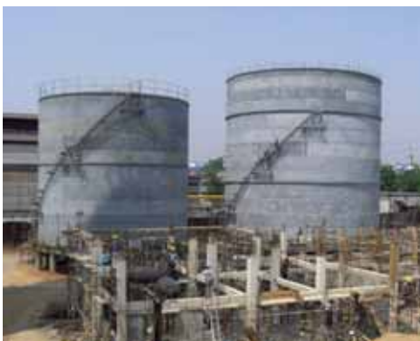
TATA Steel site, Jamshedpur
